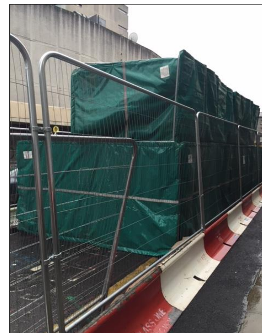
Figure 8.7 Double height acoustic blanket enclosure
