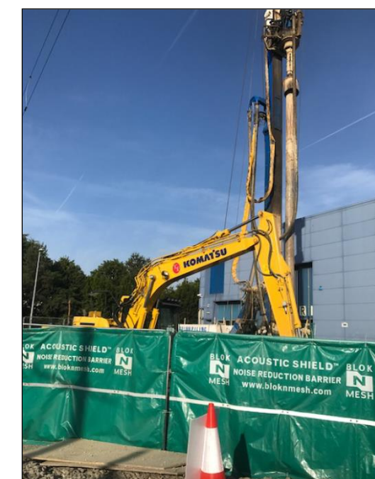
Figure 8.8 Acoustic blankets screening piling and excavations
