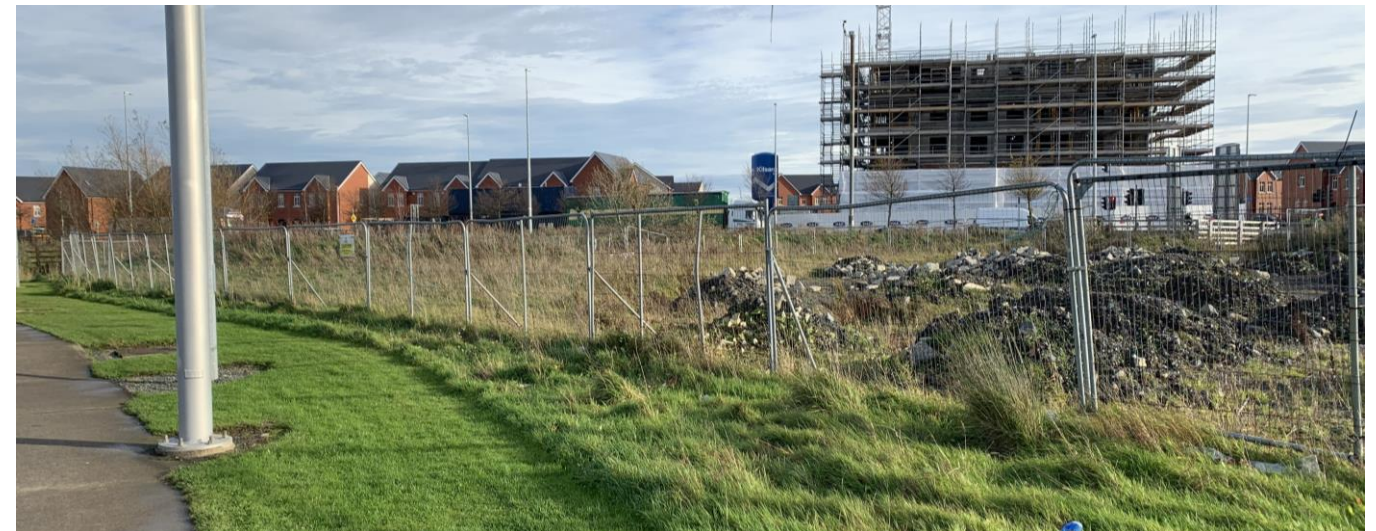
Figure 10.16: A view east from the Luas line beside the site across the future District Square towards the Citywest Village estate
