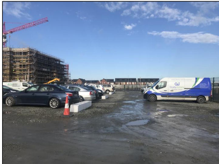
Plate 14.3 Car parking area, facing north
